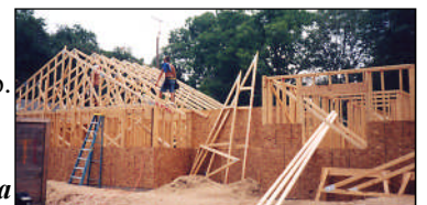
Construction of the new addition to the CODA shelter, spring 1998
